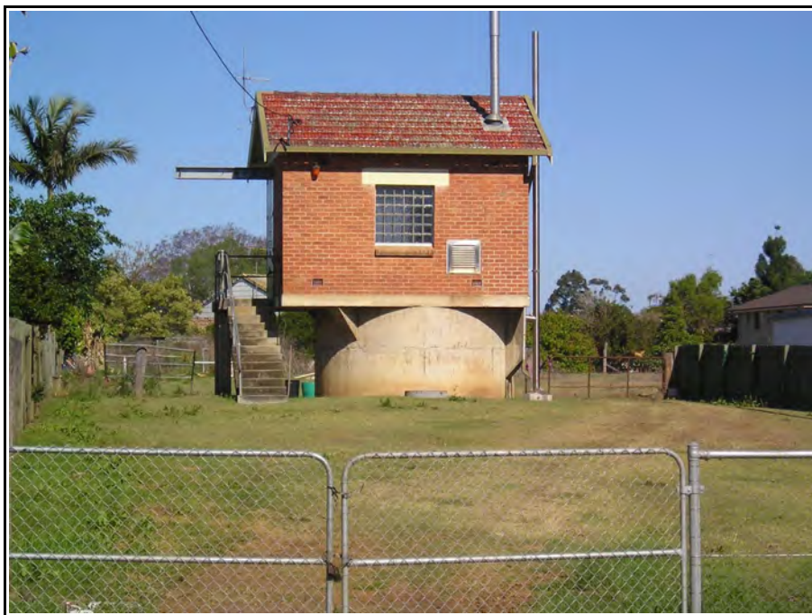
Figure 3.21 Sewerage Pump Station, c1930
