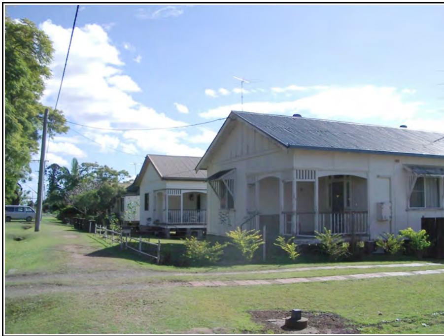
Figure 3.17 Cement Sheet Cladding, Pound Street Group
