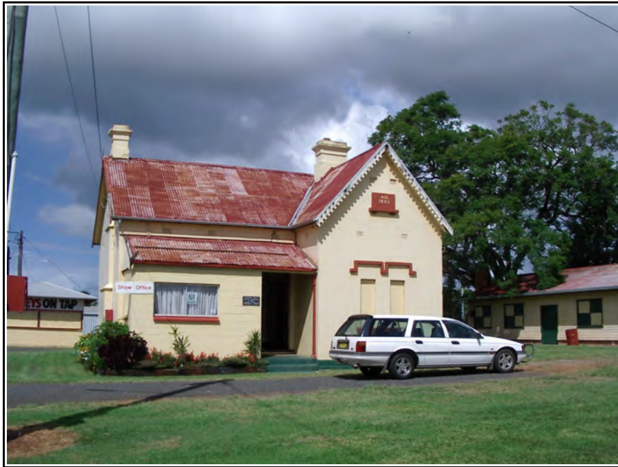
Figure 3.5 Caretakers' Cottage, Showground
