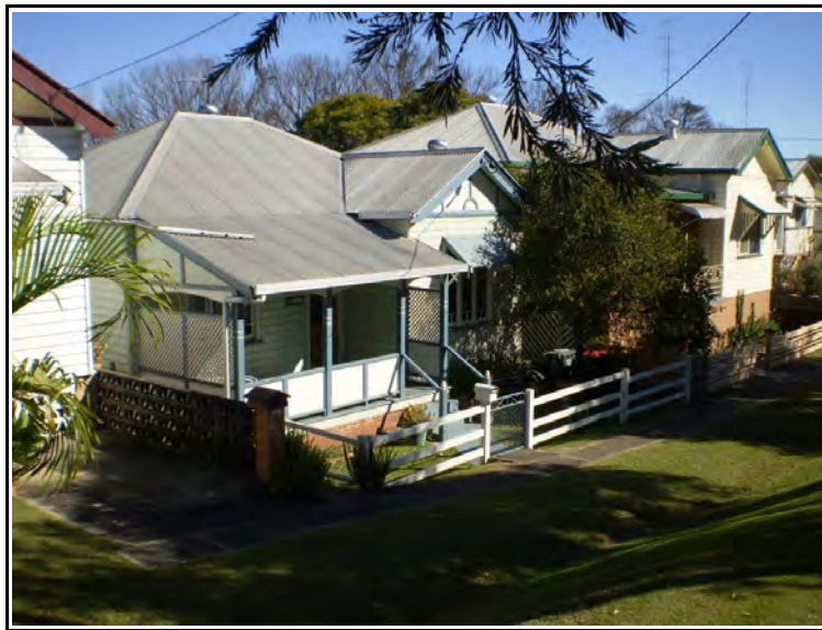
Figure 4.5 Cottage, Spring Street, South Grafton
