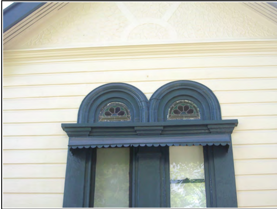
Figure 3.12 Window Mouldings, Pound Street
