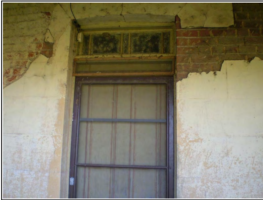
Figure 3.4 Hironnelle c1860, Swan Creek - Brickwork
