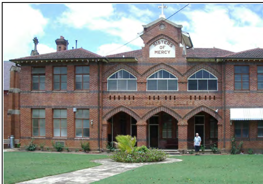
Figure 3.19 St Mary's College - St Marys' Precinct
